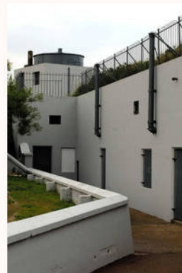
Photograph showing Outside Magazine, Blyth Battery, 2009. Reproduced with kind permission of Northumberland Archives.
